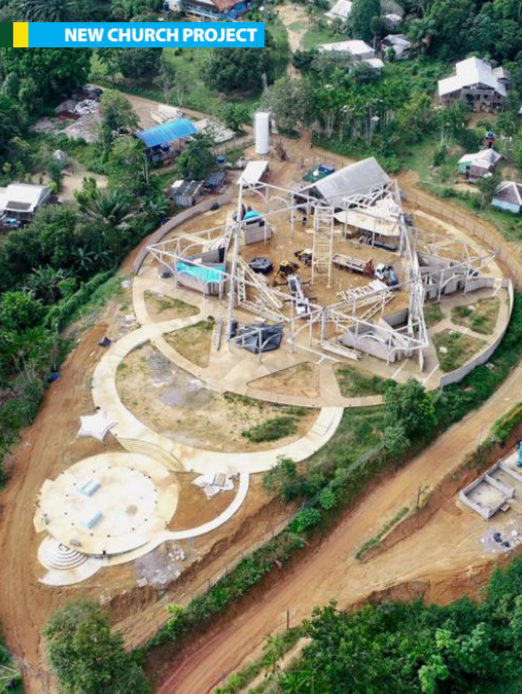
The construction continues. The sewage treatment station was installed. Currently under construction are the electrical rooms, the solar power system and the security-related structural reinforcements.
